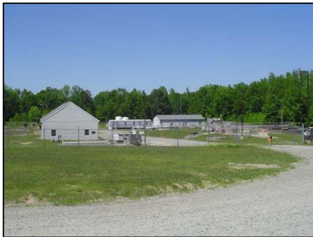
Upper Polecat Wastewater Treatment Plant
