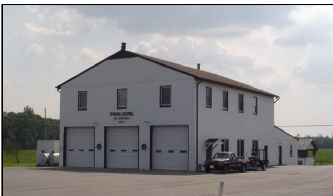
Frog Level Fire Station
